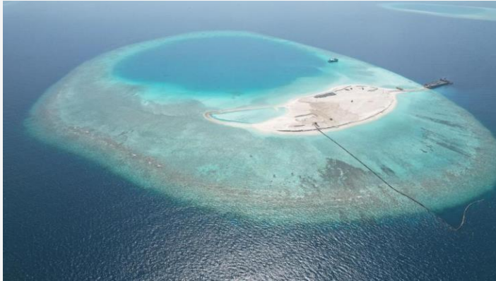
Midway of Reclamation
